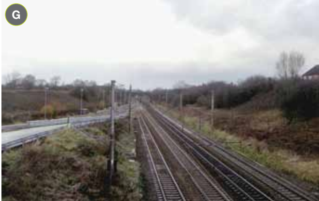
View G - View north from the existing bridge on Flag Lane highlighting the existing West Coast railway.
