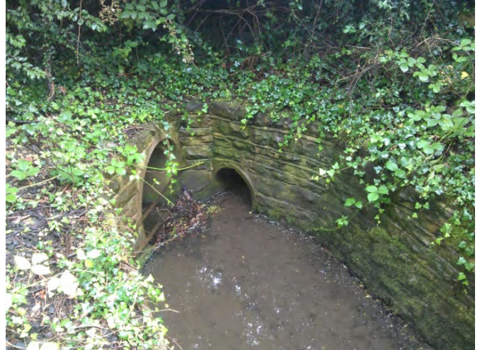
Photograph 28: View on pipes in south western corner of site.
