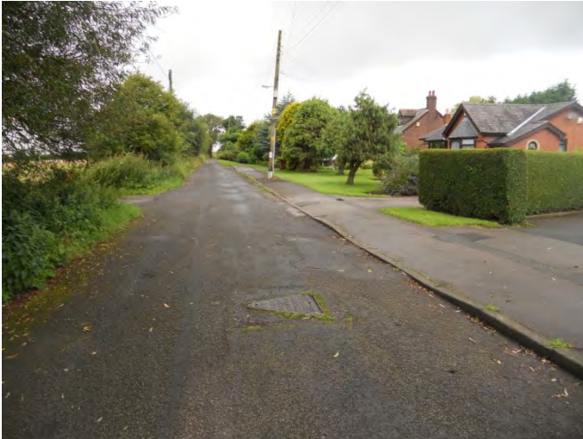
Photograph 1: View north on Banister Lane.
