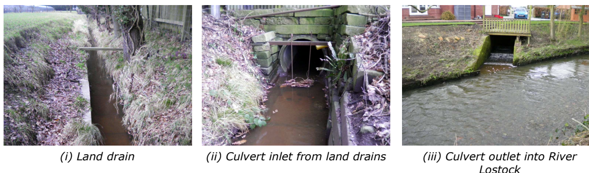
Figure 6: Land drain and culvert
