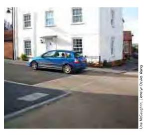
Figure 7.11 Quadrant kerbstones used instead of large radii at junctions reduce the dominance of the carriageway. This is reinforced by the placement and form of the adjacent buildings and the absence of road markings. However, note the lack of dropped kerbs and tactile paving.
