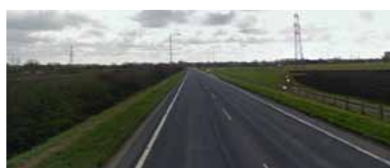
View along Flensburg Way
