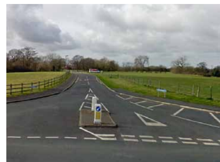
View from Croston Road along Heatherleigh
