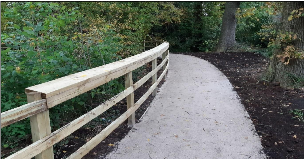
Tarn Wood, Penwortham - Replacement of a woodchip track with a stone path and improvements to the pond overflow drainage system funded by S106 green infrastructure contributions.
