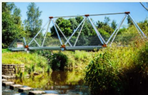
The bridge is based on a structure invented by the Scottish Engineer Charles Inglis at the turn of the 20th century. The portable bridge was specifically developed for the British Army during WW1. It was designed to enable troops, artillery and tanks to continue to advance, and to be sustained with supplies. This type of bridge played a strategically important role in 1918, enabling the Allies' sustained momentum for the advance which ended the war. Speed was vital
