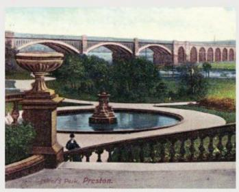
Built in 1850 this bridge originally had a series of 52 arches forming a viaduct stretching towards the *Whitehouse Junction*. Three 100ft iron arches spanned the river and at the insistence of Preston Corporation it incorporated a public footway (which still survives today!)
