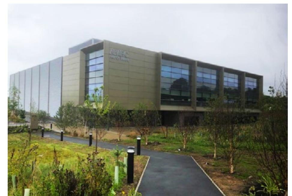
Fig. 30 - Completed landscaping within plots.
