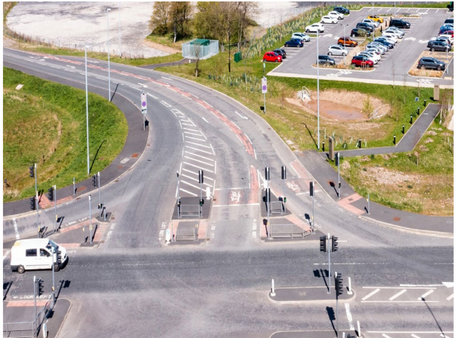
Fig. 34 - Existing photograph of the A677 junction.
