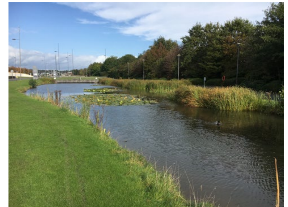
Fig.27 - Example of a Sustainable Urban Drainage System.
