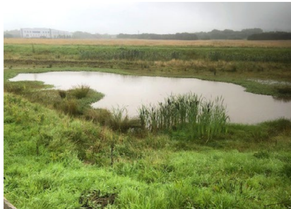
Fig. 32 - SUDS within the SEZ boundary.
